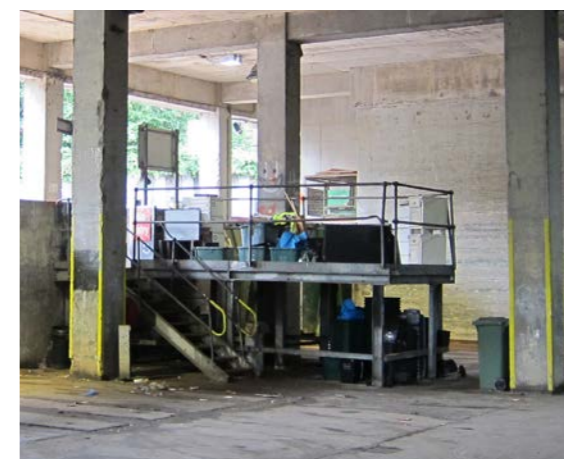
Photographs showing the existing facilities at Midland Road Recycling Centre; all by SRA Architects
